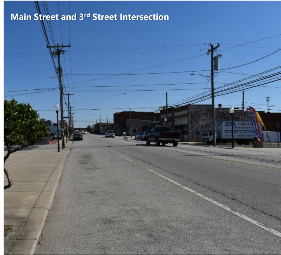
Person-level view of existing roadway.
