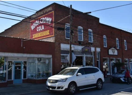
Local Businesses along Main Street
