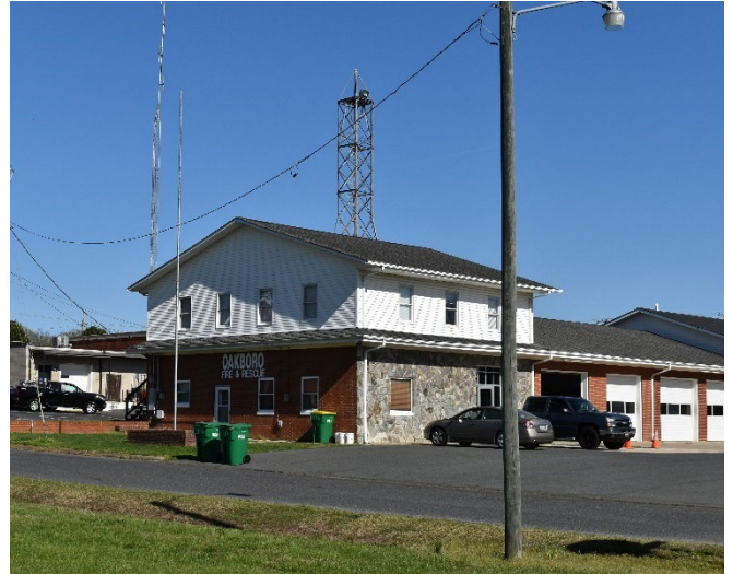
Oakboro Volunteer Fire Department Station 44
